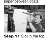
and bottom shelves, tapping in with a rubber mallet. Install the other shelves, alternating the waves with each shelf.
