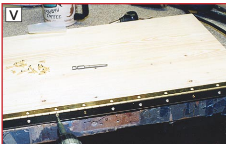
Attach Piano Hinge
