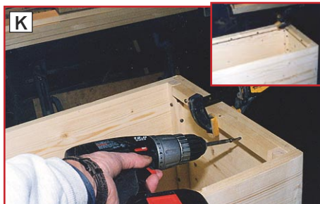
Attach Framing Cleats
