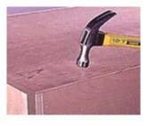
15--After checking that the case is square, install the 1/4-in. back panel with 1-in. brads driven about 4 in. apart.
