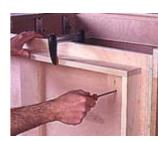
18--After assembling the kick pieces with glue and nails, clamp the base to t dresser, bore screwholes
