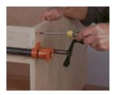
4--Assemble the case by screwing the sides to the cleats and bottom. Use clamps to hold the pieces while you drive the screws.
