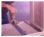
14--Install the case tracks by screwing through the horizontal slotted holes.
