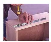
13--Fasten the drawer halves of each track to the drawer sides with screws driven through the vertical slotted holes.
