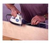
1--Heat the hot-melt adhesive on the back of the veneer tape with an iron. Slowly advance the iron with firm pressure.
