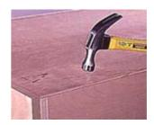
15--After checking that the case is square, install the 1/4-in. back panel with 1-in. brads driven about 4 in. apart.
