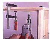
9--After gluing the edges to the plywood top, clamp the top in place and bore screwholes. Then, screw the case to the top.
