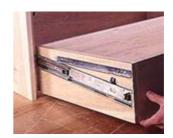
16--Install each drawer by engaging the drawer member with the hook at the back of the track. Then, lower front of drawer.
