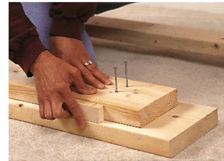
2 1/2-inch decking screws, as illustrated. The other frame end should be a mirror image of the first.
