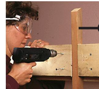
that first spacer, screw the 18 1/4-inch spacer in position (see photo). Repeat the process with the other 18 1/4-inch piece. Finally, hold the post up as a guide again, measure the remaining distance to the edge of the left leg, and cut the final spacer to fit.
