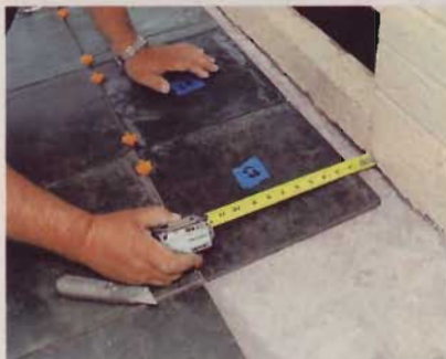
1] Do your "dry run" from front to back. This way, the narrow cut pieces will be barely visible along the back edge.
