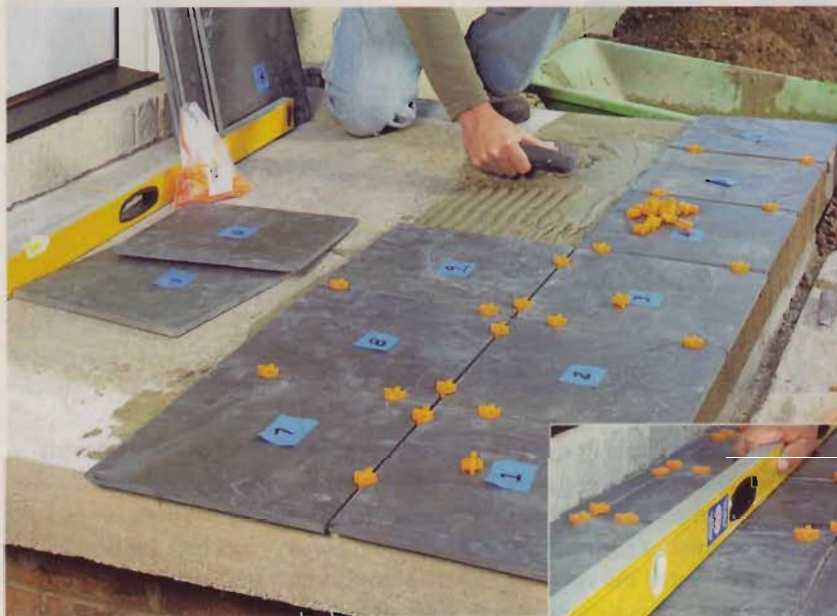
3] Lay the tiles just as in your dry run, from front to back, applying and raking out thinset as you go (above). Check each row with a level, and apply firm pressure if you need to flatten the tiles (right).
