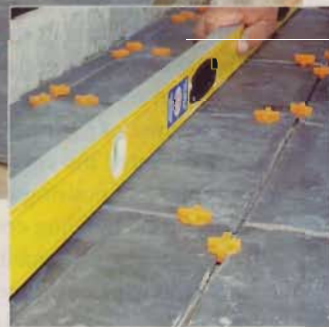
3] Lay the tiles just as in your dry run, from front to back, applying and raking out thinset as you go (above). Check each row with a level, and apply firm pressure if you need to flatten the tiles (right).
