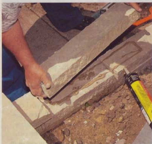
4] Before laying each stone, apply a bead of landscape adhesive, and then press the stone firmly in place to create a strong hold.
