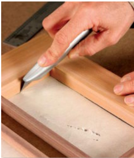
Replace major damage. If the cat decides to sharpen its claws on the paper, cut out the damaged panel from the front.
