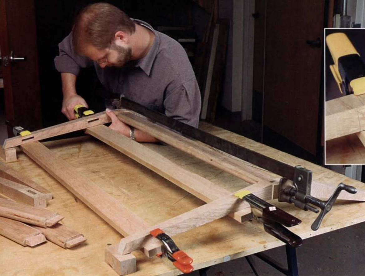
Mark tenon shoulders from the assembled back. With the rear seat rail clamped in place, make sure the assembly is square, then clamp the crest and lower back rails into place. The tenon shoulders, which are angled slightly to match the leg tapers, can be marked directly off the leg.
