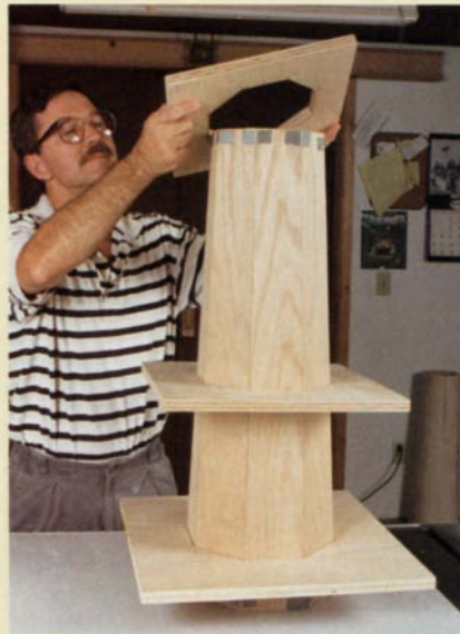
On a tapered column, plywood forms provide uniform clamping pressure. Tap them in place with a hammer.
