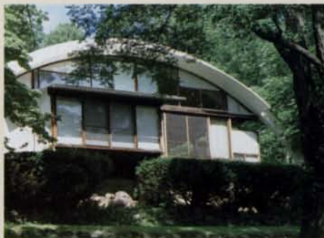
A wellspring of design inspiration. The Conoid studio is but one of the structures George built on his Pennsylvania property. The studio is named for its roof, which is a section through a cone.
