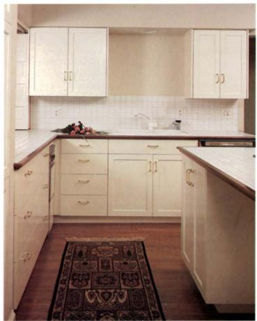
Clean, fully overlaid doors and drawer fronts give Euro-style cabinets an austere, seamless look that accrues from the efficiency of 32mm construction methods.
