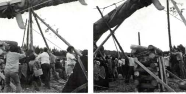
Raising the pole, June 1978. Men with small trees lashed into props steady the pole while others with long ropes heave it into position.
