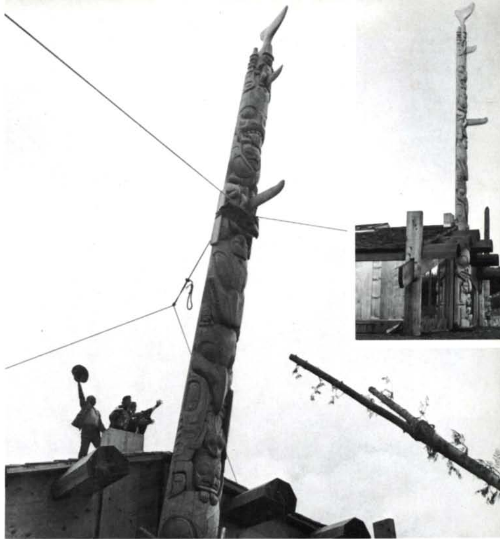
Raising the pole, June 1978. Men with small trees lashed into props steady the pole while others with long ropes heave it into position.
