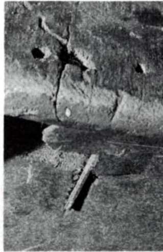
Nails and screws where there were none originally can restrict wood movement, causing checks, or splits and disfiguring holes.
