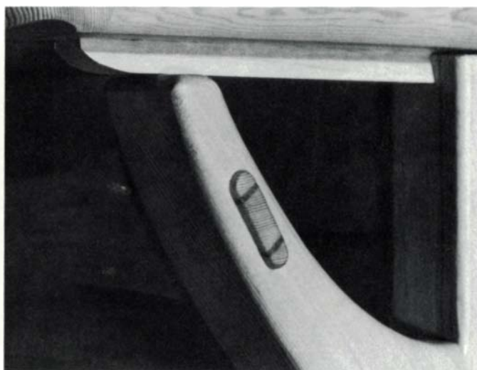
Maple slide runs in dovetail way let through leg and rests atop handle support. Below, drawer hangs from slot in apron piece that also holds divider panel.
