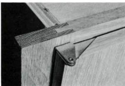
Cabinet at left has large allowance for scribing; it will be surfaced with ceramic tile. Splashboard, right, is carefully detailed.
