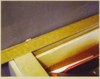
Start with the back edge. Place the strip against the back wall and see how it looks: If there is no space between the strip and the wall, that will save you some time. If there is a gap, however, you'll need to scribe the strip. Set the compass points about 1/4" (6mm) wider than the gap at its widest point. You can then run the compass along the wall and cut along the line with a jigsaw.
