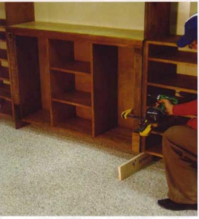
The shoe cubby and the upper cabinet to the right of the base cabinet can be reattached now. I used a 4" (102mm) spacer to establish the height of the shoe cubby.
