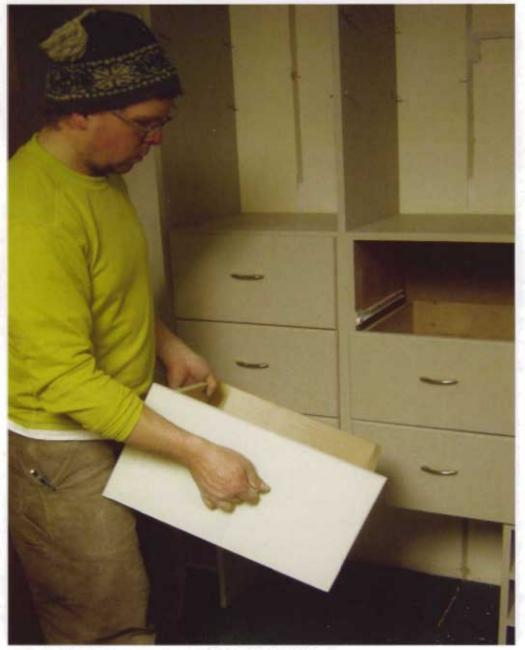
Prior to loading the parts in the van, I removed the drawers from the preassembled installation. As I removed them, I labeled them according to their position in the finished unit—it would be easy to get them mixed up otherwise. The clothes rods were easy to install. For the drywall anchors, I used 3" (76mm) toggle bolts because there weren't any studs where I needed them.
