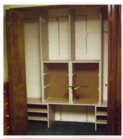
The right-hand drawer unit, with end panels attached to both sides, goes in next. Align the front edges, then clamp them together with a quick-clamp. The clamp stabilizes the assembly so you can screw it together.
