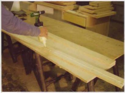
The countertops consist of <sup>3</sup>/<sub>4</sub>" (19mm) plywood that is doubled-up at its edges. Glue and screw down the 4"-wide (102mm) strips for maximum stiffness and durability. The exposed edges can be edge-banded with 2"-wide (51mm) banding when the glue has dried.
