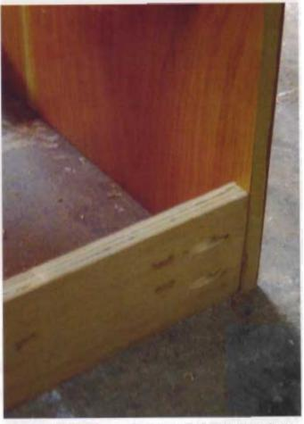
Two of the stretchers are positioned at the bottom of the unit, one at the front and one at the back, where they form a base for the bottom shelf. Place the pocket holes for the screws on the back side of the stretchers where they'll be out of sight.
