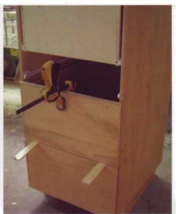
The remaining drawer fronts can be positioned using shims to create an 1/s" (3mm) gap between the drawers. Note that all of the drawer fronts can be repositioned during the final installation if necessary.
