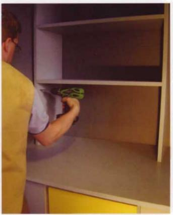
Set the bookcase directly on top of the desktop and screw it to the wall through its left-hand side.
