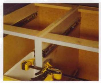
Once you've set the base into position and leveled it with shims as needed, you can set the cabinets on it. I pushed the cabinets up against the right-hand wall, then screwed them together. You'll notice that I used a quick-clamp to keep their front edges flush. This configuration left an uneven gap along the left-hand side due to some bulges in the plaster on the wall. I scribed a filler strip to fit this space.
