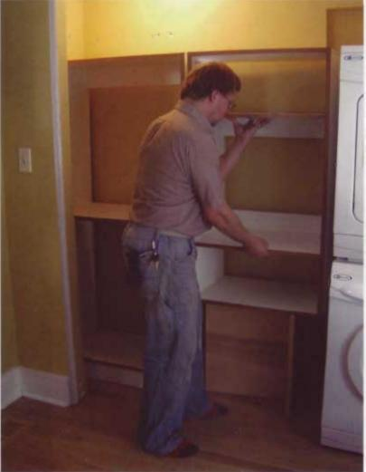
Since I performed the installation by myself, I built a temporary stand for the wall-hung cabinet. It consists of two plywood scraps that I nailed together in the shape of a T, and it provided all the support necessary to keep the cabinet in place while I fastened it to the wall.
