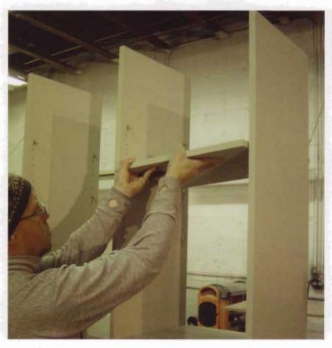
You can cut and paint the MDF shelves at any time. I like to mount them on L brackets because you can run a screw through the brackets to lock the shelves in position.
