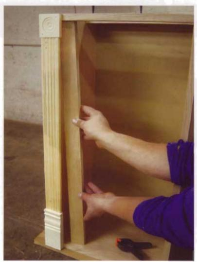
You'll notice that because the trim pieces overhang in the body of the cabinet they could be easily damaged if they're not reinforced. I put in two bracing strips.
