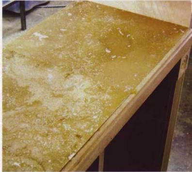
I tested the fit of the tiles and I needed to remove about 1/16" (2mm) from the edges. A quick pass over my stationary belt sander shaved it off and created a perfect fit. I waited until the rest of the project was stained and varnished before laying the tiles with construction adhesive. I coated them with stone sealer per the manufacturer's directions.
