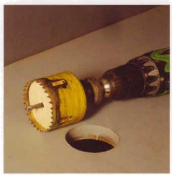
For ease of cable management, I drilled a 2<sup>1</sup>/2"-diameter (64mm) hole through the desktop near its back edge. I trimmed out the hole with a brushed nickel grommet.
