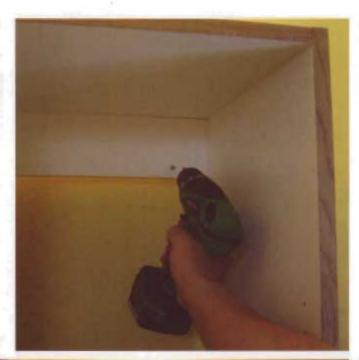
I recommend using two 3" (76mm) cabinet screws per stud.
