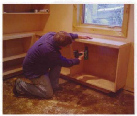
The countertops are attached to the cabinets with screws from below.
