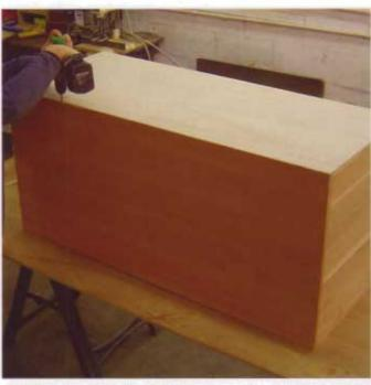
The tall drawer cabinet is straightforward: It is a four-sided box with the back screwed on.
