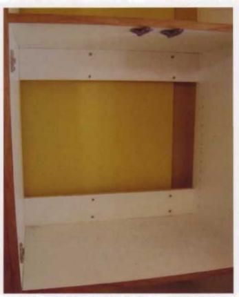
Screw the smaller cabinet to the back wall, and remove the shims and temporary support.
