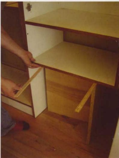
For some wiggle room, build the temporary support 1/4" (6mm) shorter than the finished height. I used shims to align the top edges of the cabinets.
