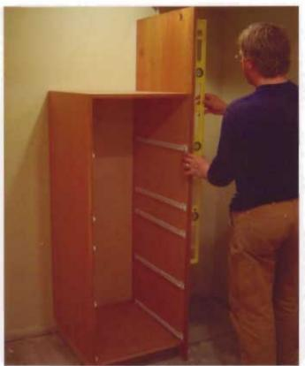
With the right-hand end panel screwed into place, position the drawer unit and make sure it is plumb and level. A few shims will help create a perfect fit. The floating shelves to the right will fit perfectly if you space the end panel 23<sup>1</sup>/4" (591mm) from the wall.
