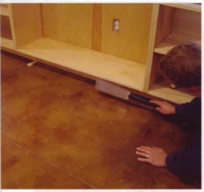
Time for the finishing touches. Cut the shims flush with the cabinet bases so the toekick trim can cover them up. I used a Dozuki-style handsaw to make guick work of this.
