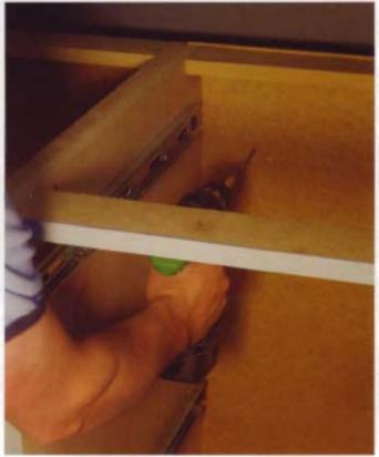
I screwed the cabinets into studs in the back wall.
