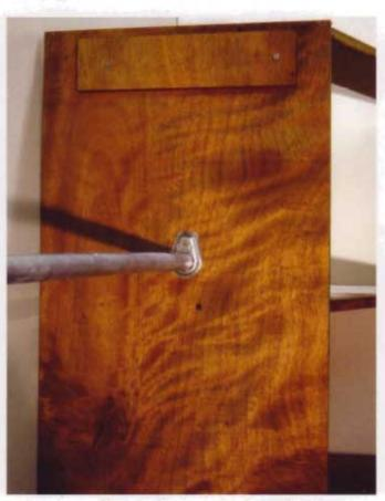
Screw the clothes rods directly onto the side panel of the corner unit. Notice that I attached a cleat above the clothes rod so the upper shelf has a place to land. The upper shelf isn't designed to support heavy objects, although you could easily reinforce it, if desired. Its main function is to provide a place to attach the crown molding.
