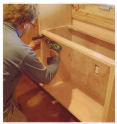
Screw the cabinets together through their sides, using clamps to line up the front edges. Then screw the cabinets to studs in the wall. A stud finder will help you locate the studs behind the cabinet backs.
