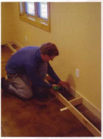
Screw the bases into studs in the back wall so they won't move around when you set the cabinets.
