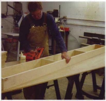
Begin by assembling the cabinet bases with glue and nails. Don't worry about the nail heads being exposed because a piece of trim will cover it later on. You'll also notice that the stretchers are inset to the fronts and backs, which is important because it allows you to use stretchers of the same length for both the sides and the interiors of the bases.
