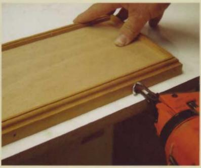
I attach the moulding with glue and nails.
