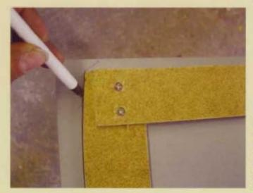
The strip should now fit against the wall; a little sandpaper will take care of any anomalies. The left and right sides are done in the same way. Once the strips fit against all three walls, you can connect them at the corners with 1/2"-long (13mm) screws. The front strip can be secured in the same way. If you take your time with the scribing and cutting, your finished desktop should drop right into place.
