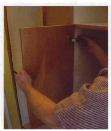
The 35mm hinges make it easy to reattach the doors on site. I generally remove them while cabinets are in transit to avoid damaging them. You may need to make a couple of minor on-site adjustments to make the doors hang evenly, but it should only take a couple of minutes.
