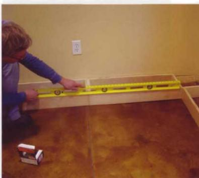
I find it easier to level the bases on a long uninterrupted run like this when they are attached. Using a 4' (1219mm) level (or a laser level, if you are so equipped), locate any spots that are out of level and shim accordingly so the entire assembly of bases reads level along its entire length.
