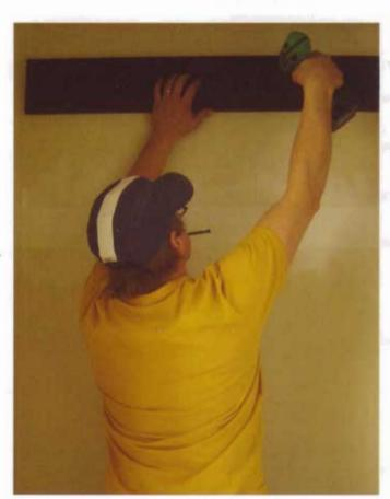
This installation was easy. I removed the old shelf and coat rod first (note the primer on the wall where they used to be). Once the primer dried, I touched up the paint to conceal all traces of the old unit. Then I screwed the back wall cleat to studs.
