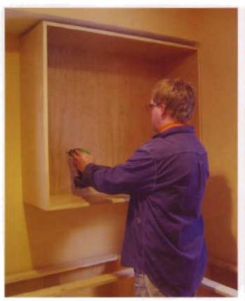
Screw the wall cabinet to the wall in six places. If you're working alone, you can prop up the cabinet on a milk crate and use some scrap wood to lift it to the right height.
