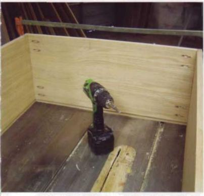
The top gets sandwiched between the sides. Locate the pocket holes on the bottom side where they are out of sight.
