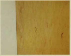
I marked the filler strip accordingly [1<sup>1</sup>/<sub>2</sub>" (38mm) from the scribed line on the top and 1" (25mm) at the bottom), and drew a straight line to connect the two marks.
