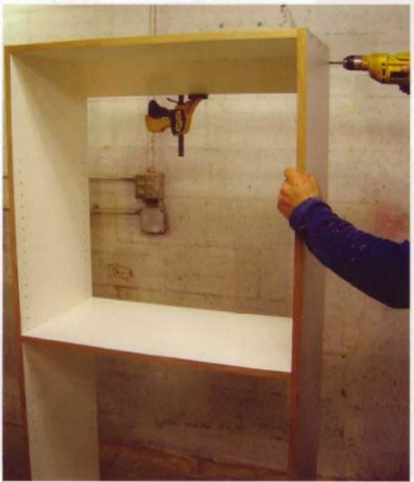
Once the fixed shelf and the top have been installed, attach the back wall stretcher in place with some countersunk screws.
