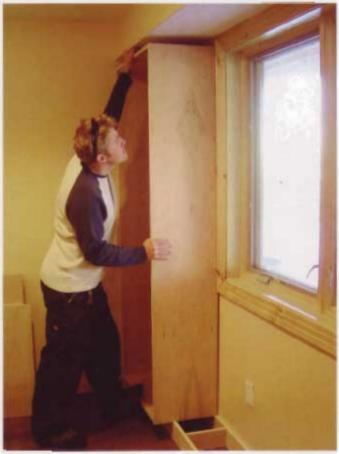
To install the cabinets, start on the left-hand side of the assembly because there's a more complicated L-shape grouping on the right-hand side which, will require the use of a filler. The cabinets at the left are positioned flush against the wall.
