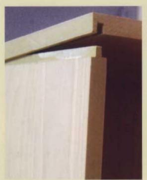
When done properly, the tongue fits into the dado without force. I lock it into place using wood glue.
