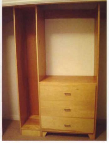
By setting up the components in the shop beforehand, I can rest assured the installation will go smoothly. Because this design is pretty simple, I'll just have to screw the components to the wall and install the clothes rods.
