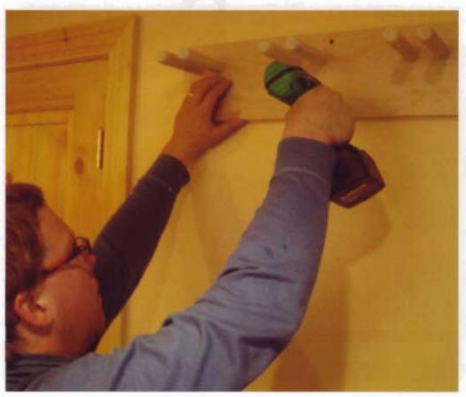
Screw the ski rack into at least two studs.
