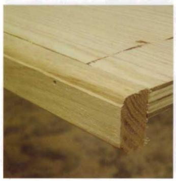
Attach a hardwood strip to the front edge of the upper shelf. It will keep the shelf from sagging over time. I used the same router bit to profile the hardwood strip as I did for the drawer fronts. Doing so provides for nice continuity between components.
