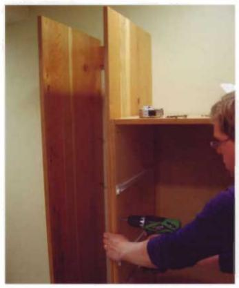
Screw the tower directly to the left side of the drawer unit. It should automatically be plumb, check to make sure it is level. Shim, if necessary, and screw it to study through its back wall stretchers.
