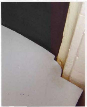
In a perfect world, the closet niche would be a precise rectangle, and you could just measure it and cut a rectangle to fit for the desktop. If you're lucky and this is the case, go for it! Otherwise, I suggest using a method for creating a template that will help you to fit a desktop or work surface into an uneven spot. (This also works great for countertops, by the way.) See the sidebar on page 62.
