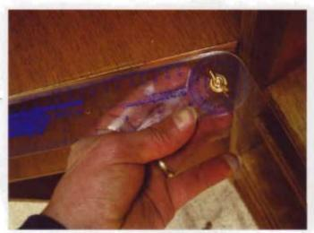
Cutting and installing crown molding is too big a topic to fully get into here, but I can at least point you to a great book on the subject: Crown Molding and Trim, Install It Like a Pro (Universal Publishers). I used an angle gauge to determine the angles where the components come together, then consulted the book to find the settings for my compound miter saw.
