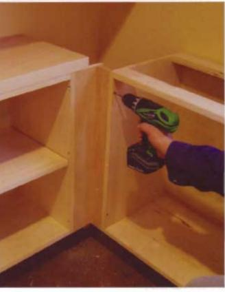
Attached the narrow filler to cabinet G, which is also screwed through the back side of the filler that is attached to cabinet F.
