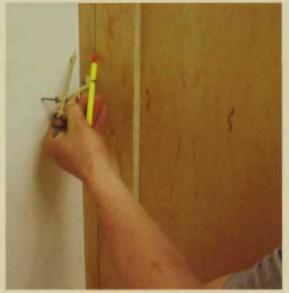
Set the compass points about 1" (25mm) apart and move the compass from top to bottom to create a pencil line that mirrors the eccentricities of the wall.
