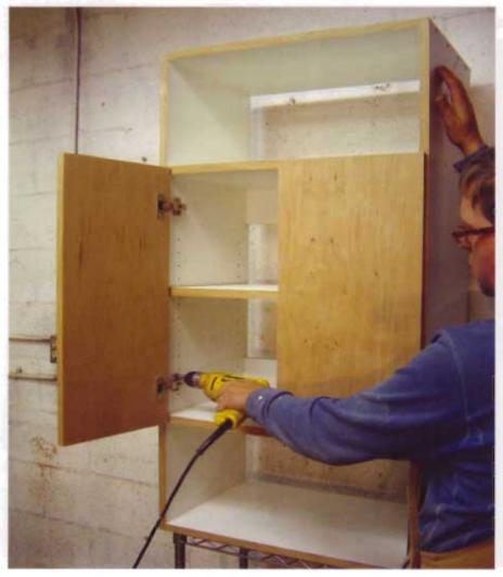
Screw the hinge cups into the doors themselves, and screw the hinge plates, with the doors attached, onto the cabinet sides. With only two doors, this is an easy task.
