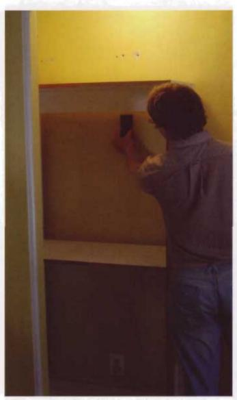
Use an electronic stud finder to locate the studs in the back wall.
