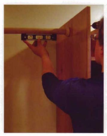
Cut the clothes rods to length, then use a level to determine the correct heights for their mounting brackets. As a finishing touch, I added some crown molding, which is visible in the photo of the finished closet. For tips on installing moldings, see Beyond the Basic Box.
