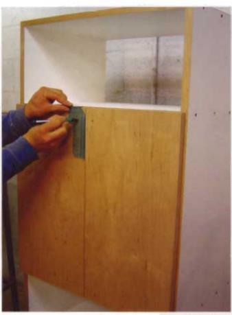
An inexpensive template (available at most home centers) makes for quick and consistent layout of the door pulls. You can see that the grain of the doors matches nicely—this is because they came from the same piece of plywood.
