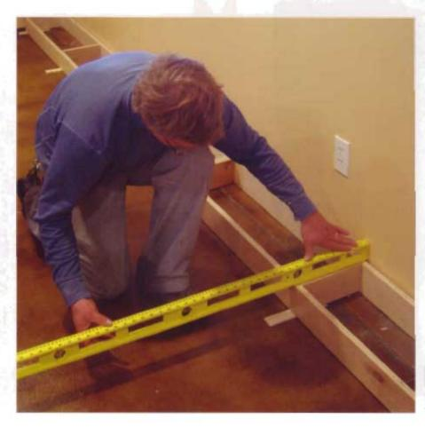
Level the bases from front to back as well. Doing so makes a huge difference in how the cabinets sit against the wall.
