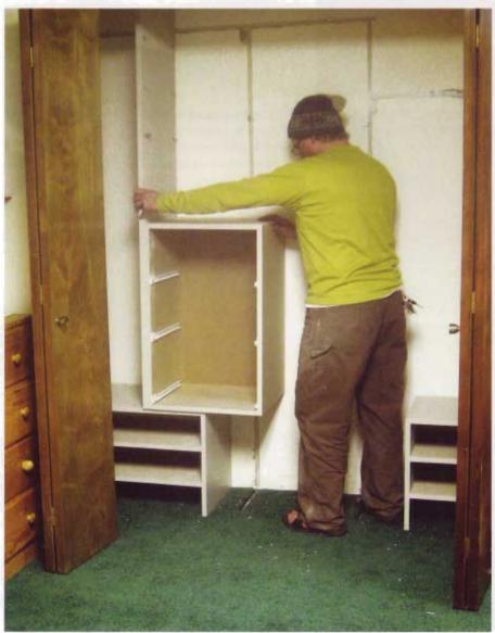
Set the left-hand drawer unit in place. I kept the end panel screwed to its side to save a step, and if I had had an assistant to help me lift it, I would've kept the entire upper assembly (both drawer units and all three end panels) screwed together. That would've saved even more time.
