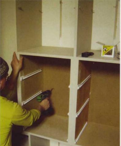
Screw the drawer units into studs in the back wall. I used 12 screws, which may be more than necessary, but better safe than sorry.
