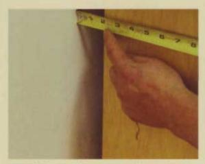
To fit the filler to the gap, measure the gap at the top and bottom of the cabinet. In this case, it was about 11/2" (38mm) at the top and 1" (25mm) at the bottom.
