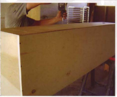
The 1/4" (6mm) plywood back is attached with screws and glue.
