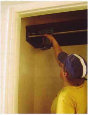
I next screwed the side wall cleats into studs. Once I dropped the shelf into place and screwed in the coat rod, I vacuumed the closet and set the cabinet into place.
