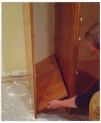
The bottom shelf is placed in the tower and secured with construction adhesive.
