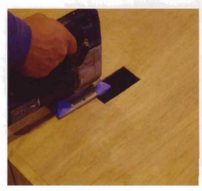
Cut holes into the cabinet backs where needed for electrical outlets. A jigsaw does the job quickly and neatly.
