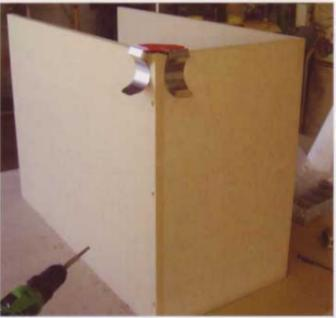
Cabinets A,B,C and D all go together the same way. I used through screws, since the sides won't show and there's no need to conceal the joinery. Just be sure to predrill and countersink for the screws. I also recommend setting the screws a few inches in from the corners if you use MDF, since it tends to split if screws are driven into its edges near a corner. And don't be stingy with the glue—the adhesives will provide a lot of the strength in this case.
