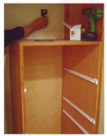
Screw the drawer unit to the back wall. A stud finder will make it easy to locate the studs.
