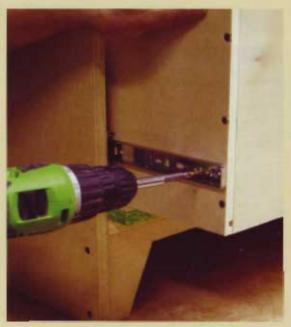
Affix each slide with three screws, then flip the cabinet over and repeat the process on the opposite side.
