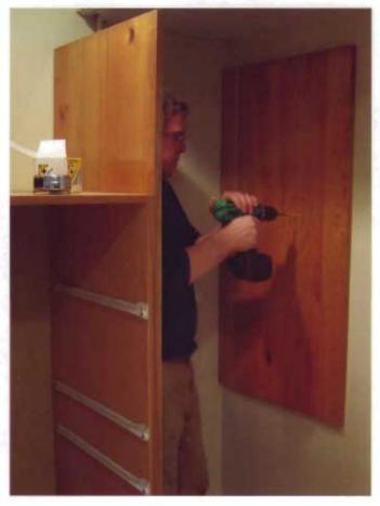
Screw the short end panel into studs in the right-hand wall to create a space for the floating shelves. Place a level on top of the left-hand end panel and across the gap where the shelves will go. When the bubble is perfectly centered, mark the wall accordingly. This indicates the height at which to place the short end panel. Don't simply measure up from the floor—it could be inaccurate due to variations in the height of the flooring.
