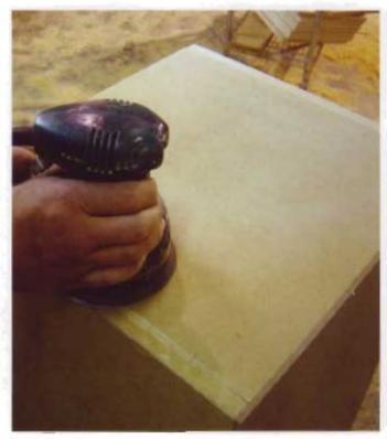
When the glue has cured, remove the clamps and sand the joints flush on the top. This will be visible in the finished closet, so a smooth, uniform surface is ideal here. Any gaps can be filled with putty and resanded. I used 60- and 80-grit paper to sand down large discrepancies.
