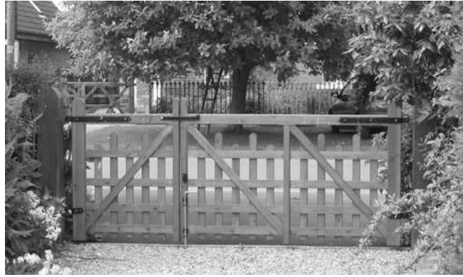
Fig. 6.2 Modified field gate to include personnel access
