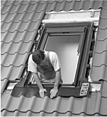
Fig. 3.39 Fixing the flashing
