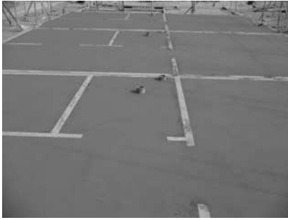
(a) Soleplate in place, used to provide a floor screed. Notice the provision for service pipes
