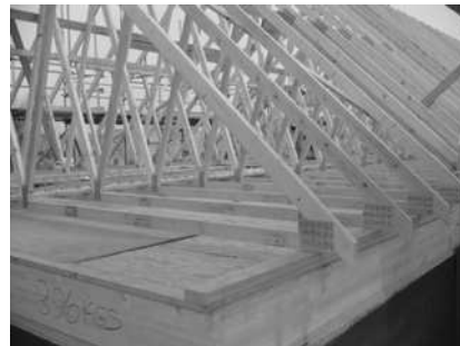
(d) Roof trusses pre-assembled over ground floor slab – prior to being lifted up in place
