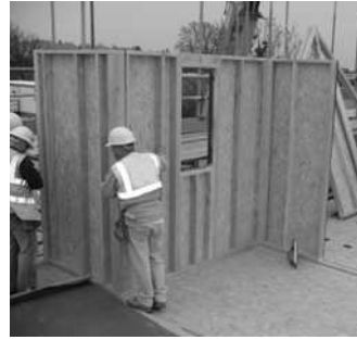
(b) Exterior corner panels being erected
