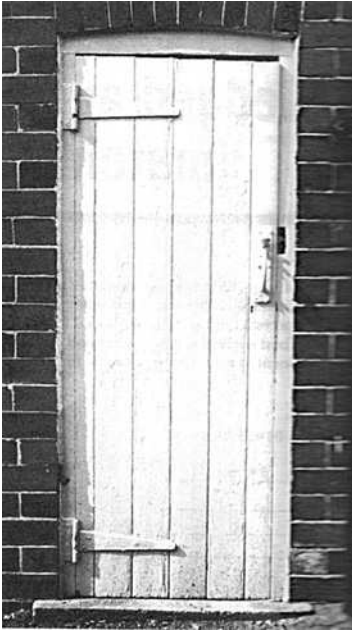
Fig. 4.4 Example of door sag (missing 'sag bar')
