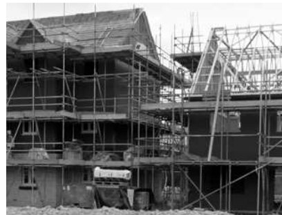
(f) Exterior cladding in progress on left hand construction
