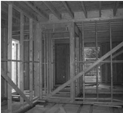
(c) Interior studwork showing temporary bracing for stability
