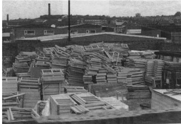
Fig. 3.55 How not to store window frames on site
