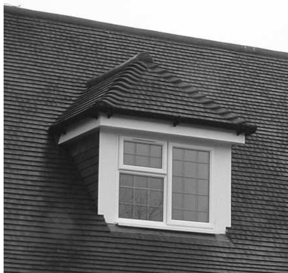
Fig. 3.42 Dormer window with hipped ended pitched roof
