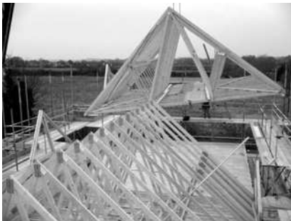
(e) Part of pre-assembled roof being lifted and lowered into position
