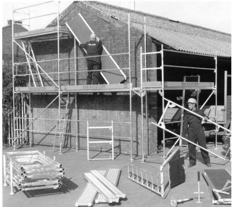
**Fig. 10.17** *Frame system scaffold*
