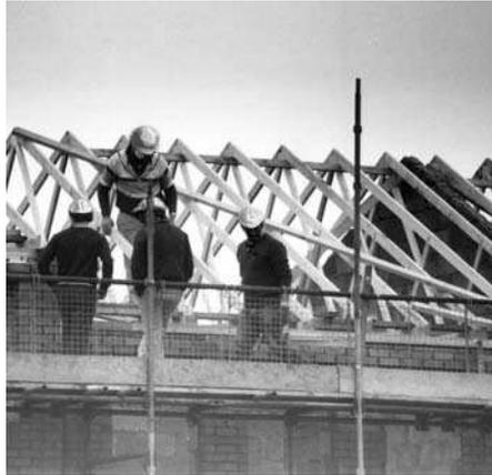
**Fig. 8.28** *Trussed-rafter roof being erected*
