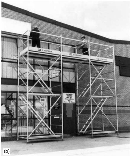
Fig. 10.20 (a) Static tower with stabilising outriggers; and (b) two static towers linked together
