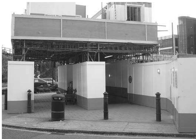
**Fig. 2.12** Hoarding encroaching onto footpath with site offices above
