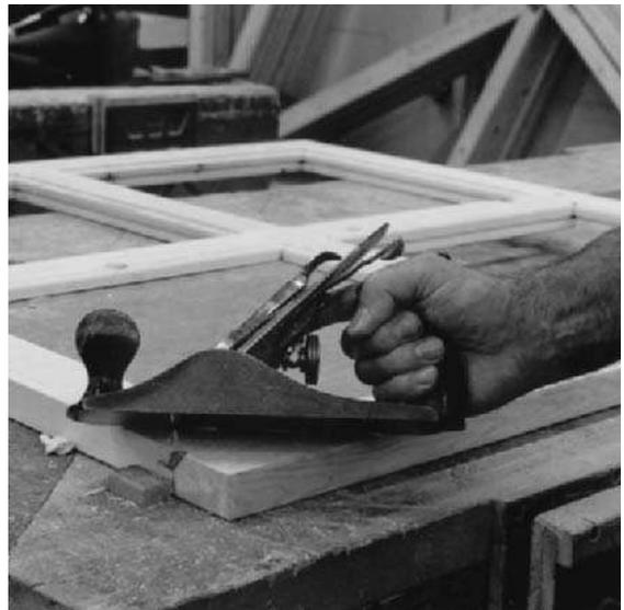
(d) Testing a corner joint for flatness by tilting the plane – notice the light showing between the edge of the plane sole and the surface of the timber, indicating that, at this position, the surface is hollow
