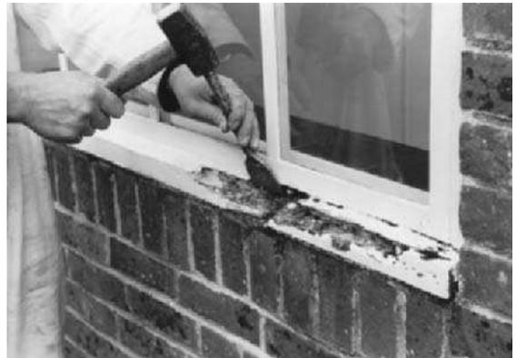
**Fig 2.10** A typical wet-rot location (window sill) – with kind permission of Rentokil)
