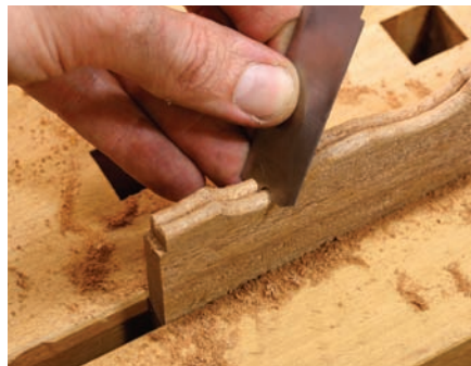
Scrape your profile. This gorgeous little double-arch mould was a breeze to make. I made a scraper out of a leftover piece of saw blade. Five minutes with a chainsaw file and voila! This drawer blade follows the contour of the drawers above and below it.
