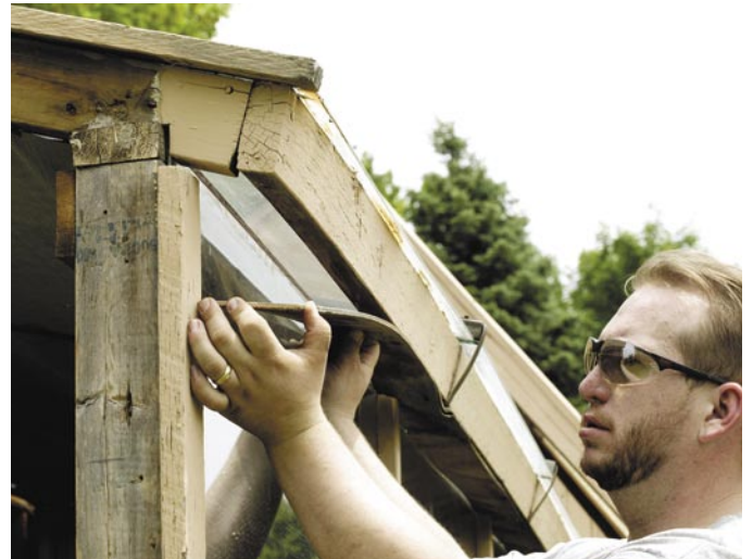
The space at the top of the window wall is opened by removing the soffit panels. It is when green wood is first introduced that this venting of moisture-laden air is necessary. Later in the drying cycle, the soffit is screwed shut to increase temperatures in the kiln, while moisture is dissipated through small cracks in the structure's simple construction.
