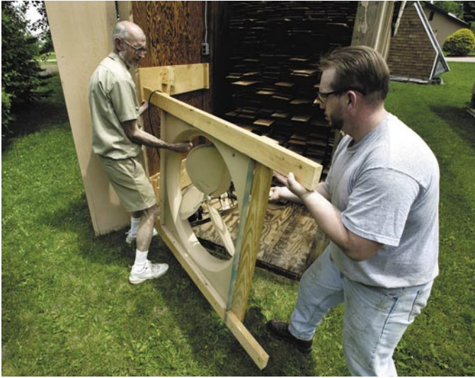
Before loading, the end of the kiln is opened by a hinged door panel and unscrewing a 4'-wide main panel. The 30" fan is being removed to give access.
