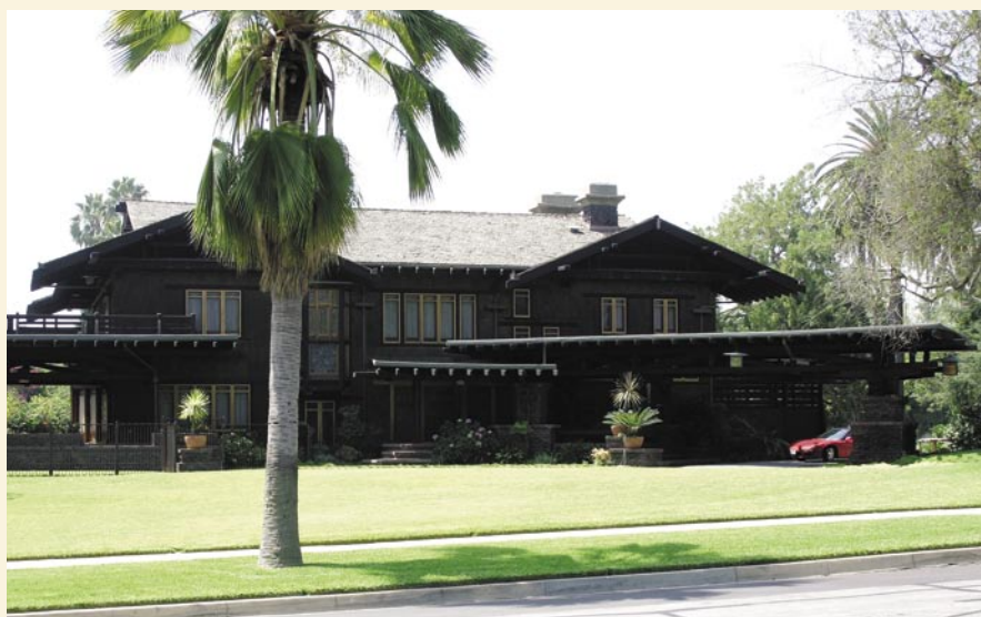
The renovation of the Blacker house is complete. Many of the original furniture pieces have also been reproduced, and more are planned.
