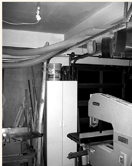
A single 50-watt halogen spot light on the ceiling augments the workshop's fluorescent lighting and provides focused brightness at the band saw blade.
