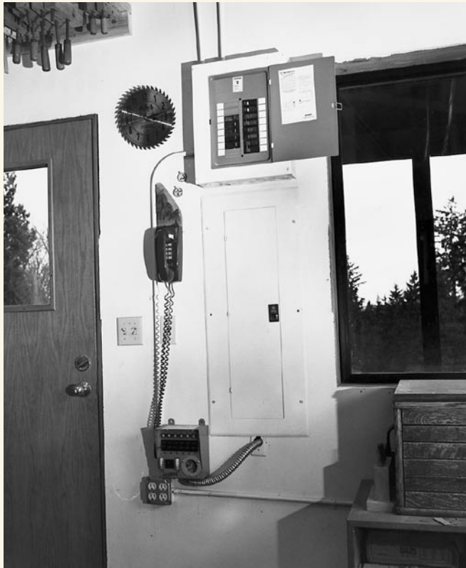
This subpanel cover is removed for a better look at the breaker switches and wiring.
