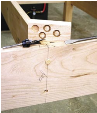
Use a tapered countersink and #8 x 1 1/4" screws to attach the center support, then fill the holes with matching face-grained plugs.
