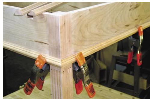
Miter the corners of the moulding and use a thin bead of glue. Too much glue and the result might squeeze out onto the aprons, causing finish problems.
