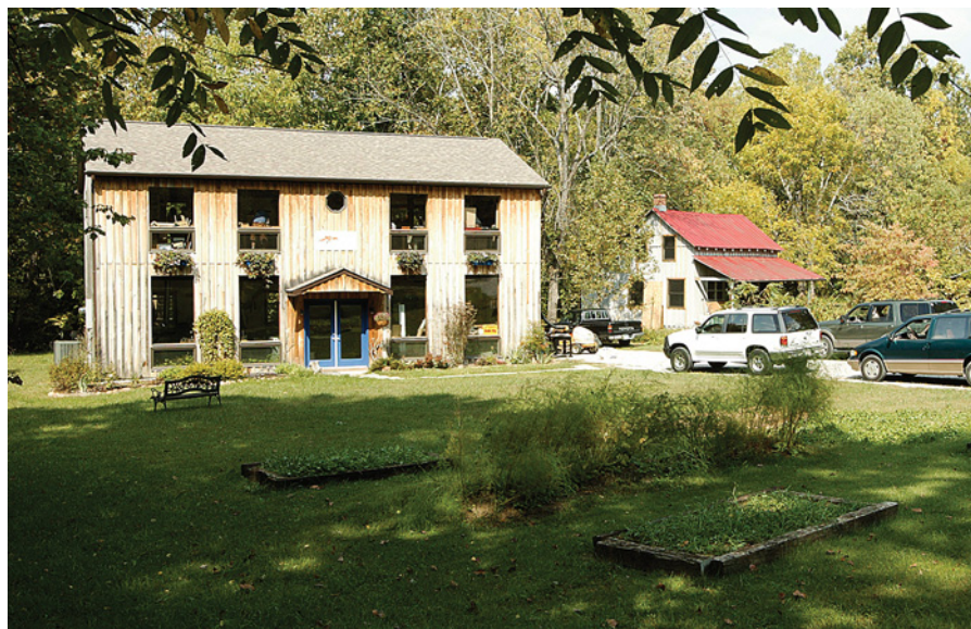
Mehler’s two-story school is constructed and situated for maximum energy efficiency, with large, south-facing windows for maximum natural light, thick walls for good insulation and high ceilings to disperse excess heat. Next to the two-story shop sits a 19th-century Kentucky box house, which has been rehabbed with all the modern conveniences. While visiting instructors get first dibs, the cozy house is available for student rental.
