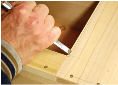
The junction of the horizontal and vertical beads must be completed with a little paring chisel work.
