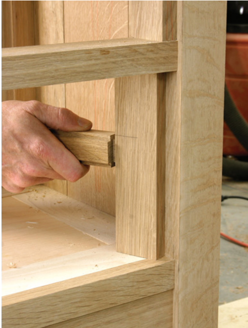
The drawer runners have a tenon on the front end that fits in a mortise in the stile. These are placed in position before the stile is glued in place.
