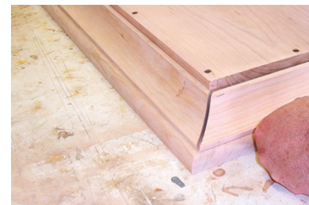
The cove moulding is attached to the torsion buildup, below the top. I used a shop-made cove for this piece.
