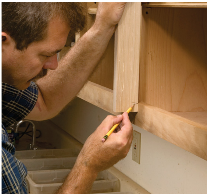
For an exact fit, mark measurements on pieces using mating parts, not rulers. Here you can see I'm marking a stile for a cabinet.
