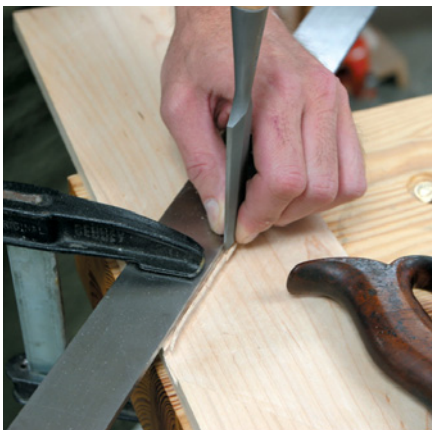
Mark your 45° angles using a knife. Clamp a steel straightedge against the knife line and chisel away your waste. Or pare to the line freehand.
