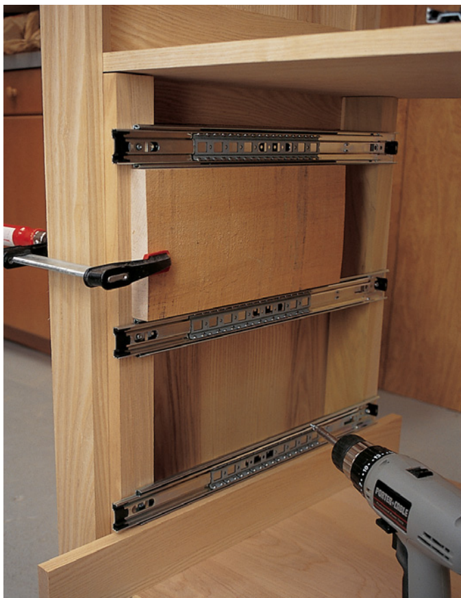
Use spacers to hold the hardware parallel to the cabinet bottom. The spacers also ensure the hardware will be located at the same height on both sides of the cabinet.
