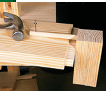
To accurately position the hole for the brass nut shown in the photo, build a simple jig like the one shown here using 1/2" dowel, a scrap of wood and a nail. The nail is located where you want the center of the brass nut to go (top). Insert the dowel into the hole in the rail and tap the nail (bottom). Now drill a 1"-diameter hole there and your joint will go together with ease.
