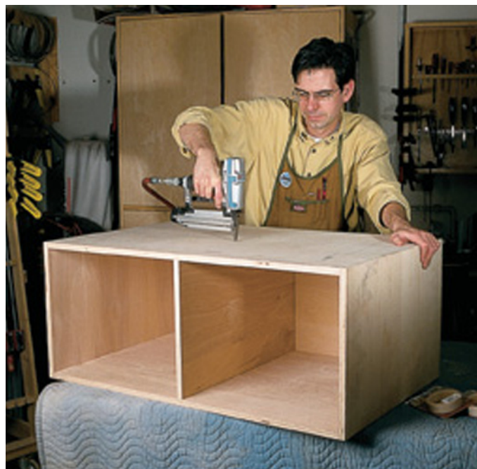
I nailed the divider in place in the toolbox so I could check and double-check its position before fixing it in place.
