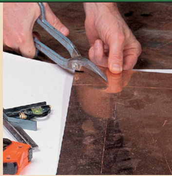
After drawing a line from a corner to the intersection of two score lines, cut out one of the triangular shapes from each corner using snips.
