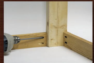
Assemble flush & corner joints
