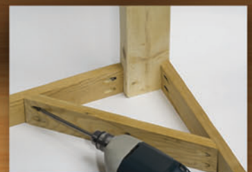
Assemble angle joints
