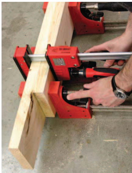
Almost an instant tenon. Leave the tenons way overlong. They'll be mitered to size after you excavate your mortises.
