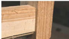
Not too shabby. The finished joint looks surprisingly good to me.
