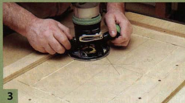
3 Rout a rectangular hole in the center of the sub-top. Make a series of shallow passes until you've cut all the way through. Place the solid surface top on the sub-top.
