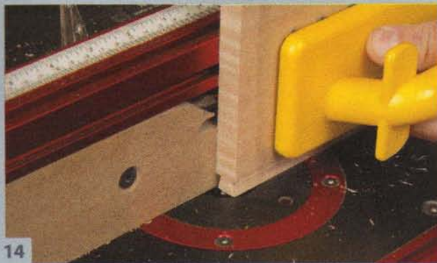
14 Rout the tails . Use a push block to hold the workpiece tight against the fence and to keep your fingers out of harm's way.
