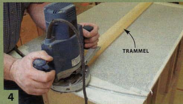
4 Rout an arc on one end of the solid-surface top using a trammel fastened to the router's base.
