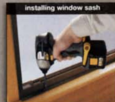
installing window sash
