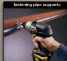
fastening pipe supports
