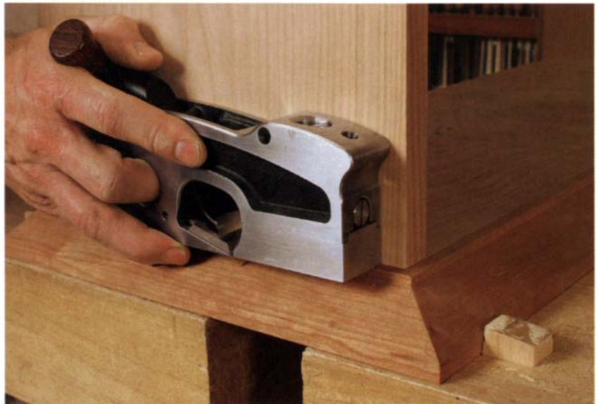
Plane moldings flush. The top edges of the front and side base moldings were slightly misaligned. Gochnour uses a shoulder plane to get the parts flush.
