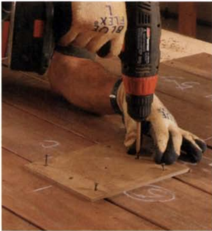
Pivot block prevents marring the top boards. Drive screws between the top boards to hold the block in place. A pivot pin in the trammel engages the center hole in the block.
