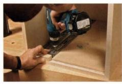
A trick for installing slides. Working off the centerlines of the drawers and slides, Schleining uses a spacer panel to set the distance between the slides and the cabinet bottom. A small block sets the distance from the front edge.
