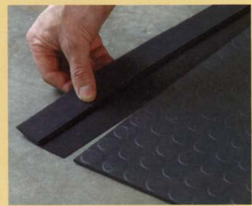
A clean finish. Some manufacturers offer edge strips, which are snapped on or glued into place.
