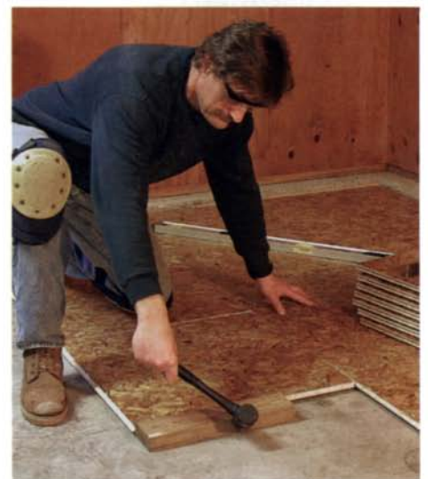
Shop flooring for covering concrete, p. 50
