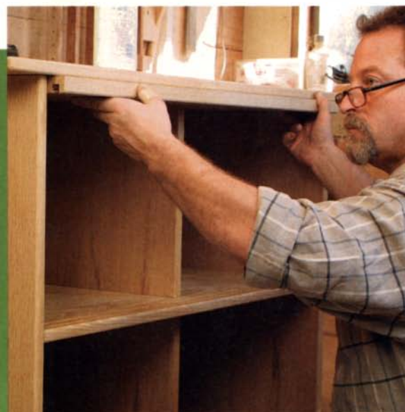
Install the upper track. Be sure that the grooves in the track are aligned with the corresponding grooves below.
