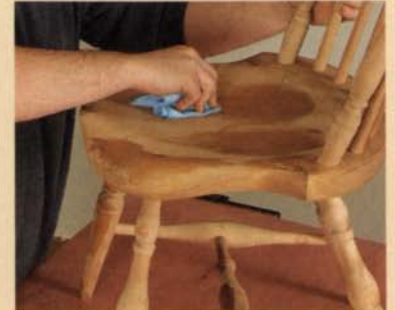
Wax the wear areas. Rub paste wax onto those areas of the chair that get rubbed the most during normal use.
