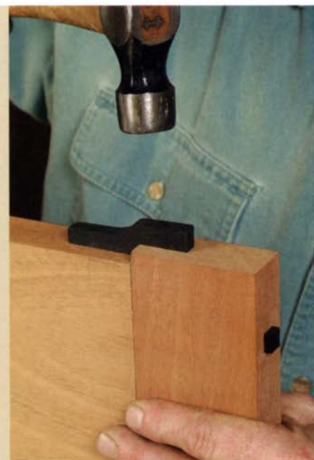
Apply the ebony plugs and end caps. Glue the ebony end cap only to the tabletop panel so that it can move freely in the breadboard end.
