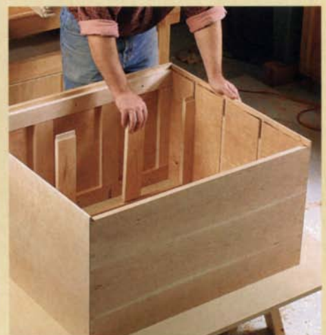
Installing the drawer frames. Begin by gluing the front stretchers in place (left). Then flip over the case and insert the runners into the front stretchers, applying glue only at the front tenons (right). Finally, glue the back stretchers into place.
