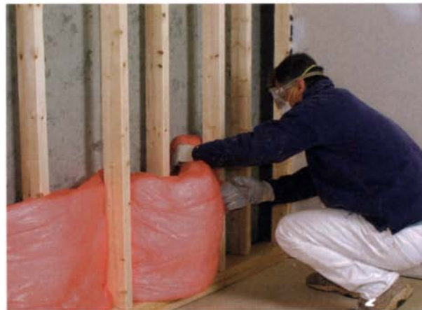
Meant for heat but good for sound. Standard fiberglass batting, designed and traditionally used as a thermal insulation, also happens to be a pretty good sound dampener. A second layer of drywall will decrease substantially the level of sound that penetrates the structure. Stagger seams to ensure an airtight bond.
