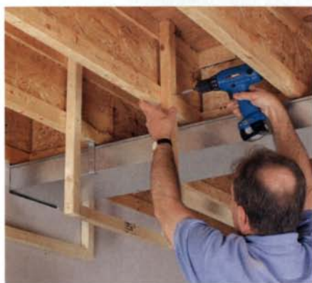
Cover the duct with a framed opening. Simple 2x3 frames assembled at the workbench are easily attached to floor joists with screws.
