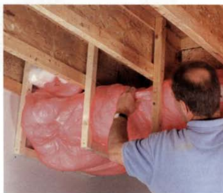
Stuff the airspace with thermal insulation. Fill the airspace around the duct with good-quality fiberglass insulation. Higher R-values dampen noise more effectively.
