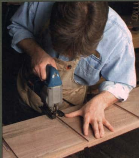
Cut away the wood you don't need. Housed lap joints require you to remove some wood from all of the pieces being joined. In the verticals, remove most of the waste with a sabersaw.
