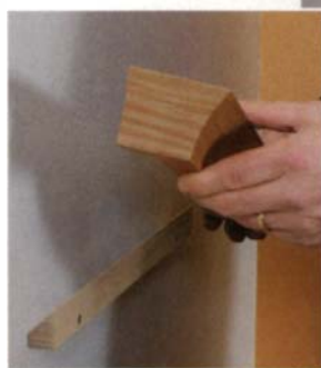
A French cleat bears the weight. The base engages with the wall cleat, and the cabinet sits atop the base. The case requires only a single screw at the top to hold it securely to the wall.
