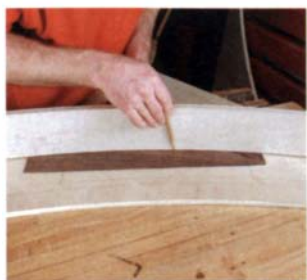
Use the apron as a template. O'Malley cut the beading material in three sections.
