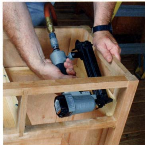
Tack in the side blocking. Finish the interior of the drawer-guide installation by attaching the side blocking.
