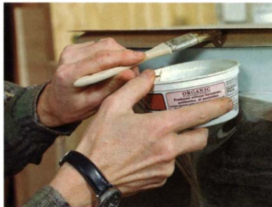
After the first pressing, the edge is prepared for gluing. First, spread plastic resin glue around the edge and deep into the crevice.
