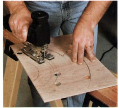
Cut out the opening. To achieve a nice radius, drill \frac{3}{4} -in.-dia. holes in the corners before cutting out the opening with a sabersaw.
