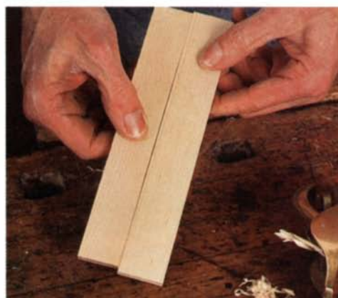
Cut the cleats to fit the grooves, then plane their bottom edges slightly concave. Later, when they are pulled down into their grooves, the cleats will make firm contact at both ends.
