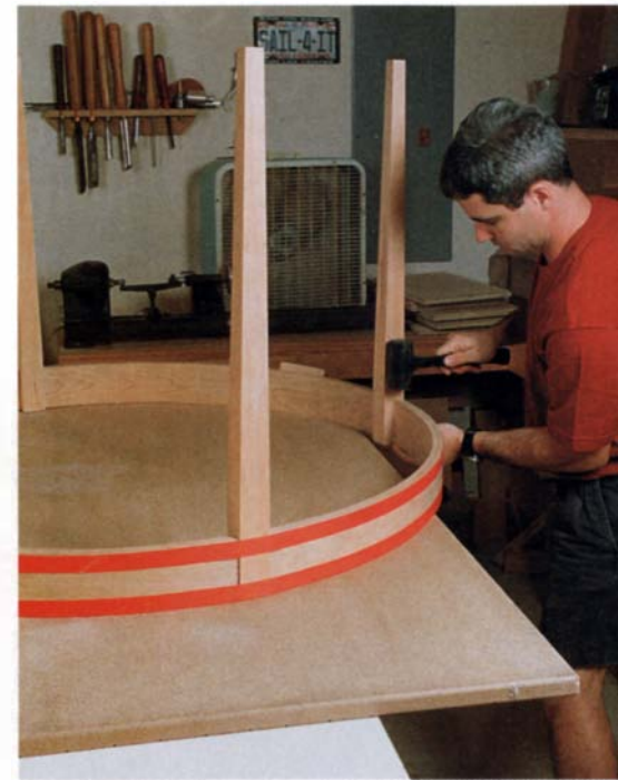
Tweaking the alignment. By hanging one leg joint over the edge of the worktable, the aprons and legs can be drawn flush together with a deadblow hammer before the clamps are fully tightened.
