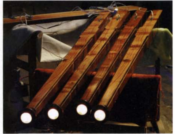
The lights are connected to one master switch. The wires exit near the bottom of each post through holes drilled below the bed-rail hardware.
