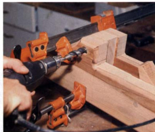
Delicate drill work. If the hole for the treadle pivot pin is not accurately drilled, the whole clamping system can be thrown off. Drill by hand from both sides or set up an extension table and use a drill press.
