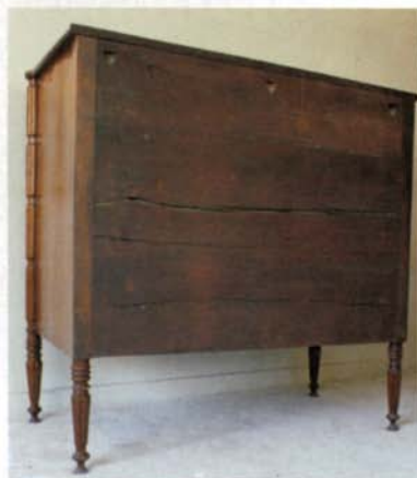
Fastened back boards split, too. The back of the chest with the split sides is screwed to the top and nailed to the bottom of the chest. A paneled back would have fared better.
