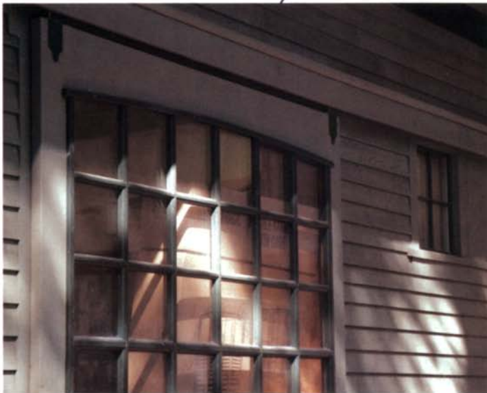
A door to ease the load. A large door on a barn-door track slides open to make awkward loads more manageable. The author opted for a glass door to keep the shop well-lit.
