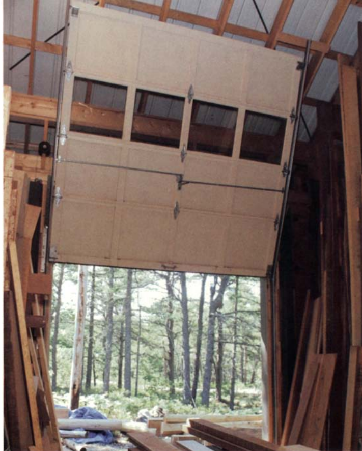
Door stays out of the way. The author modified a regular garage door; otherwise, it would have made moving and sorting boards in the vertical storage area difficult. He hacksawed a kerf in the tracks the door rides in, then straightened them and oriented them almost vertically. Counterweighting the door makes it easy to open.
