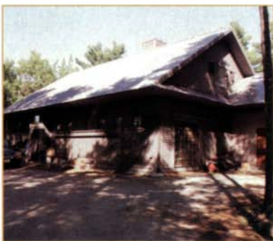
Door stays out of the way. The author modified a regular garage door; otherwise, it would have made moving and sorting boards in the vertical storage area difficult. He hacksawed a kerf in the tracks the door rides in, then straightened them and oriented them almost vertically. Counterweighting the door makes it easy to open.
