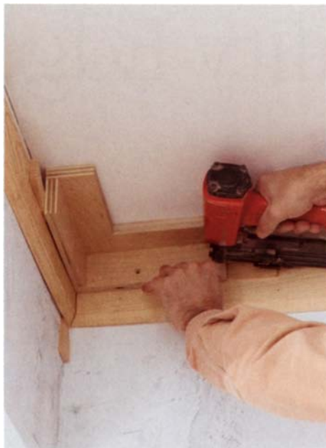
Shims help create square corners. During installation, pine shims fill gaps in out-of-square corners at walls and ceilings. Once the brackets are screwed into place, trim off the excess by scoring the shim with a utility knife.
