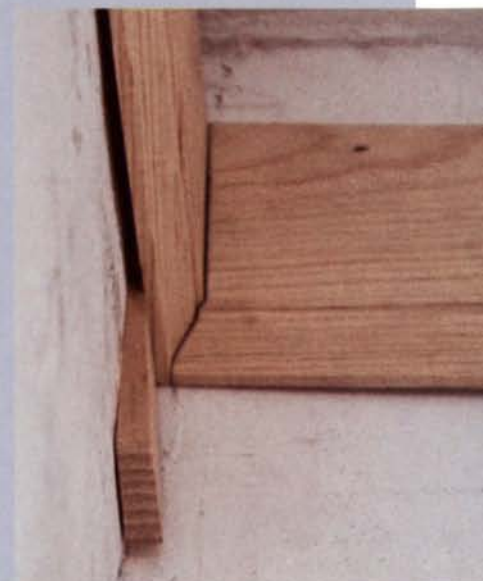
Installed and shimmed
